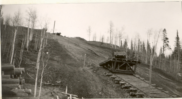
Hoist pulling a loaded sled up from the river flat to the bench where the Phoenix Lumber Co. mill is situated, Clearwater Forest, 1923
